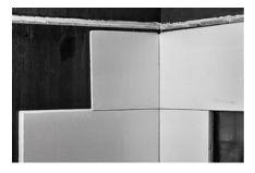
Protect the membrane from mechanical damage by means of thermal insulation or protective slabs.
